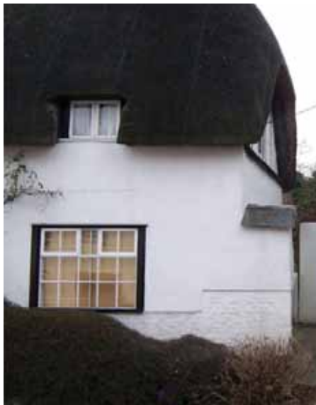
C - Church Street, Durrington Relevant design elements: - Timber casement windows - Render and whitewash - Thatched roof
